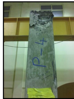
Figure (13) P-4 Concrete Cracks
