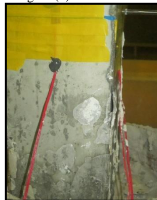
Figure (10) P-3 Flange Buckling
