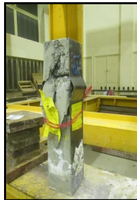
Figure (4) P-1 Concrete Crack
