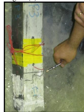
Figure (11) P-2 Failure zones
