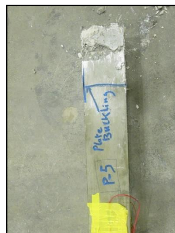
Figure (15) P-5 Concrete Cracks
