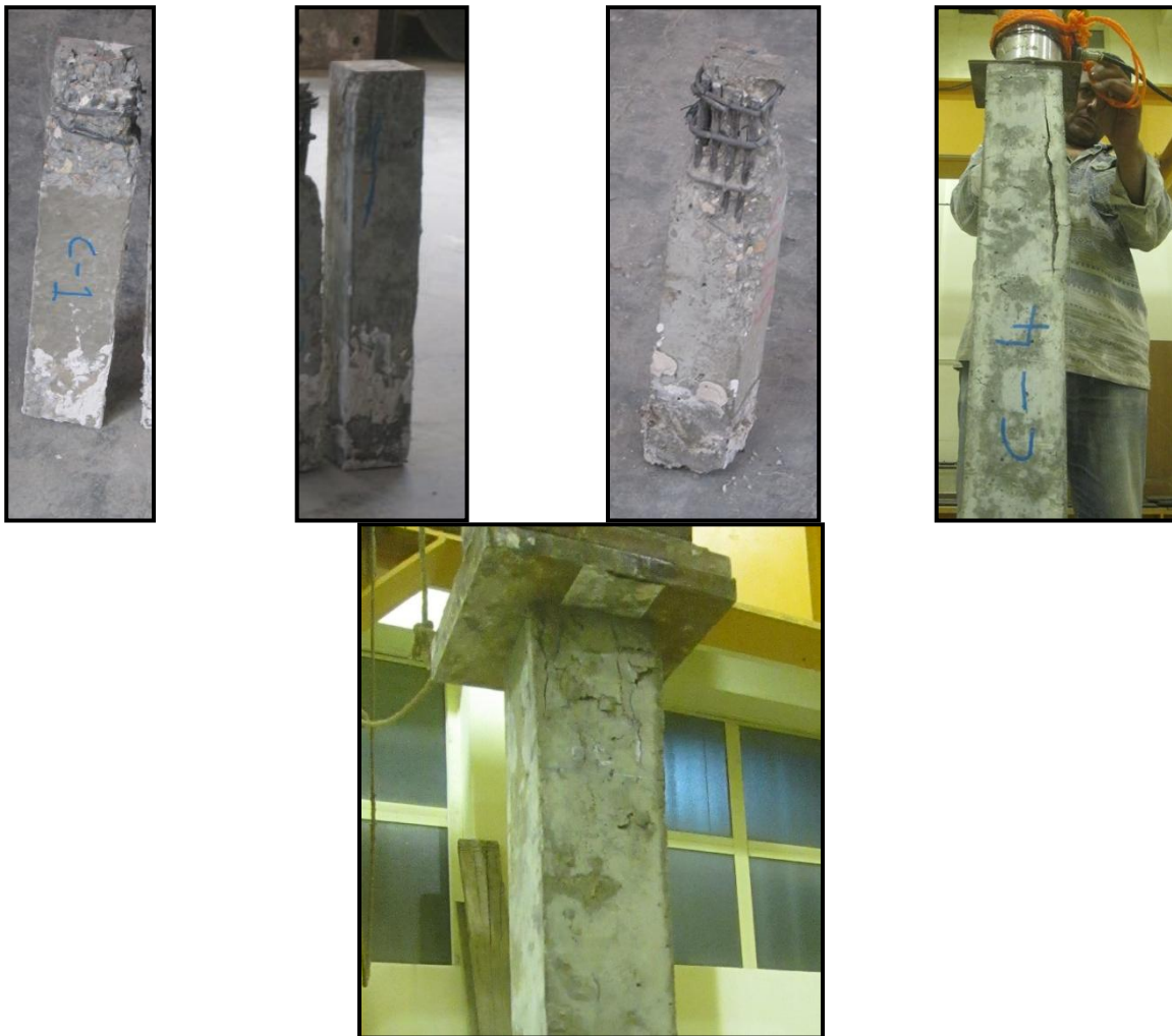
Figure (17) Reinforced Concrete Specimens after Failure
